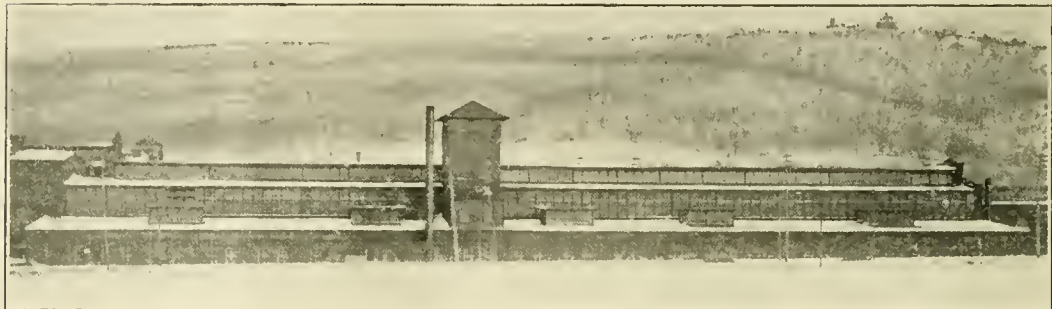
BOILER SHOP, FROM HIGH GROUND TO THE WEST. RIVETING TOWER AT THE CENTER. SHOWS THE LARGE AMOUNT OF GLASS IN ROOF.
